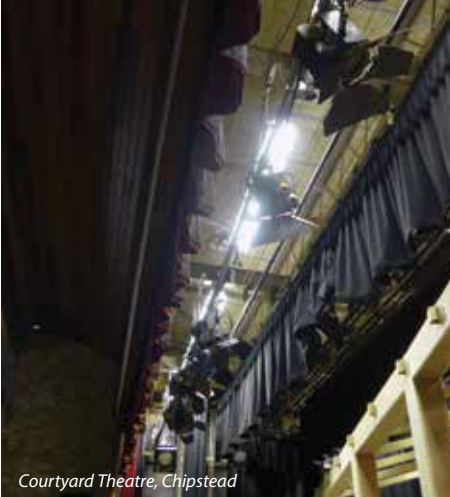
Courtyard Theatre, Chipstead
