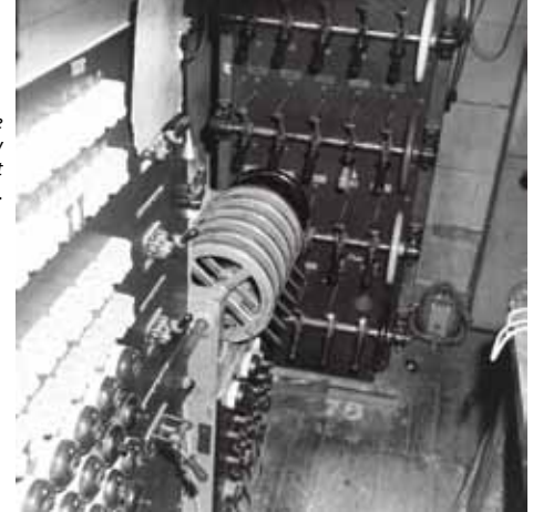
Worthing Pavilion c.1968. Permanent bracket handle dimmers in the background with temporary 12-way interlock (centre) and fuses for the permanent installation on the left.
