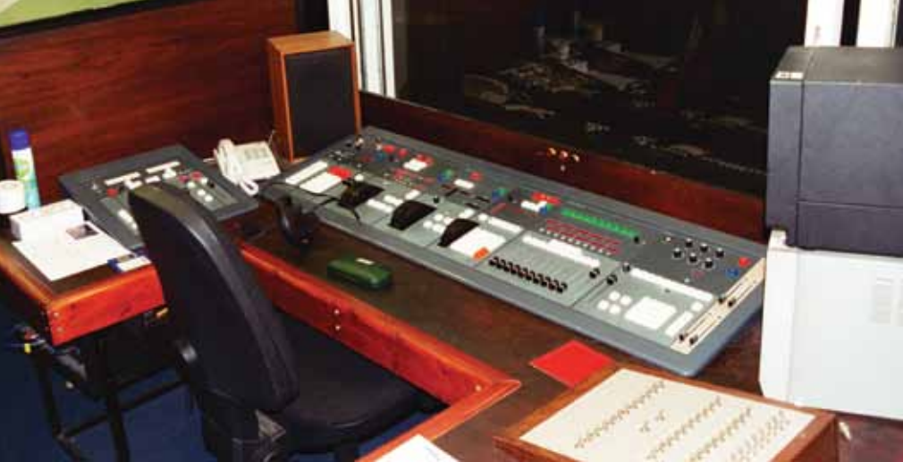
Royal Northern College of Music, Opera Theatre, Manchester. Galaxy Nova in the control room c2004. The desk was originally installed in the Edinburgh Festival Theatre, then used for touring before installation in the RNCM.
