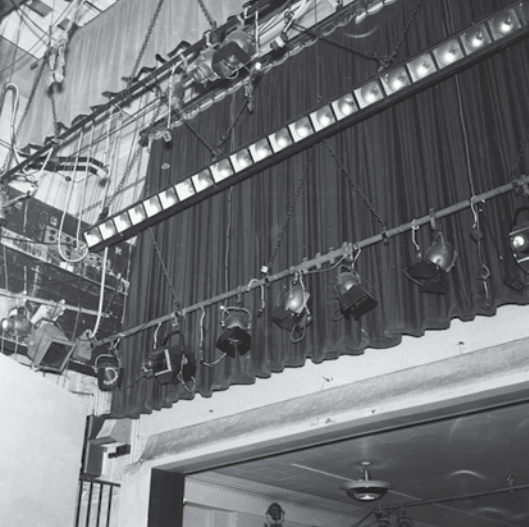
Imperial College, London c1964. Overhead rig for a play and Strand Electric SR control (right).
