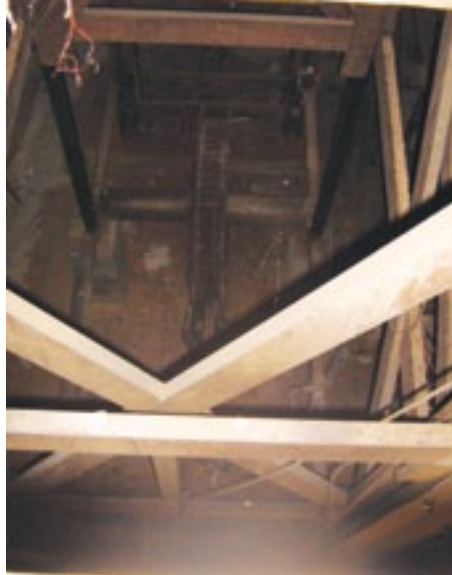
A view through a trap sub-stage showing part of the original trap mechanics.
