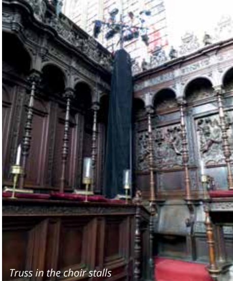
Truss in the choir stalls
